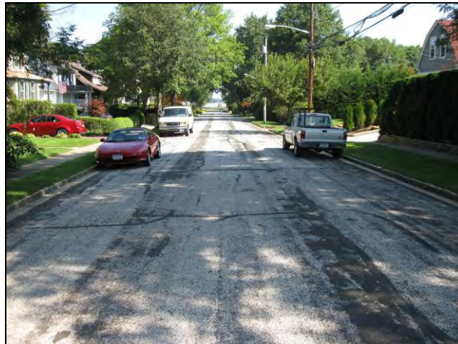
Views of Ships Point Lane residences, which is a potential candidate for a green streets retrofit.
