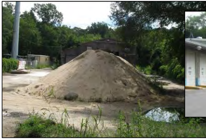
Uncovered materials storage
