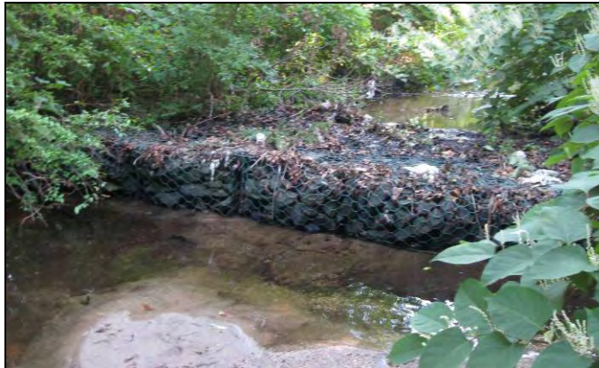
Gabion wall along reach CSB-04
