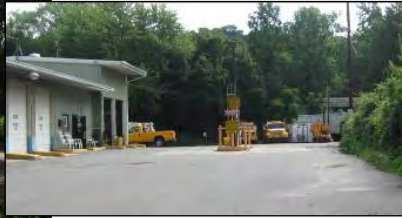
Uncovered fueling station
