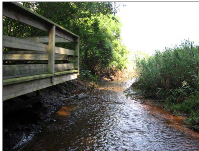
Impacted buffer along reach CBS-01 near the Cold Spring Fish Hatchery property.
